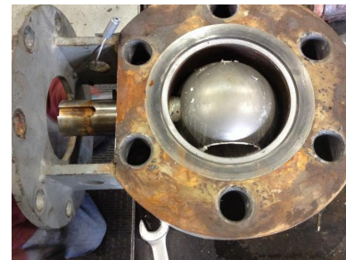
Application-specific design allowed this MOGAS ball valve to perform flawlessly for more than six years.
