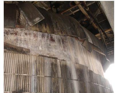
Leaking water from a competitor's valve caused damage to the coke drum's thermal insulation.
